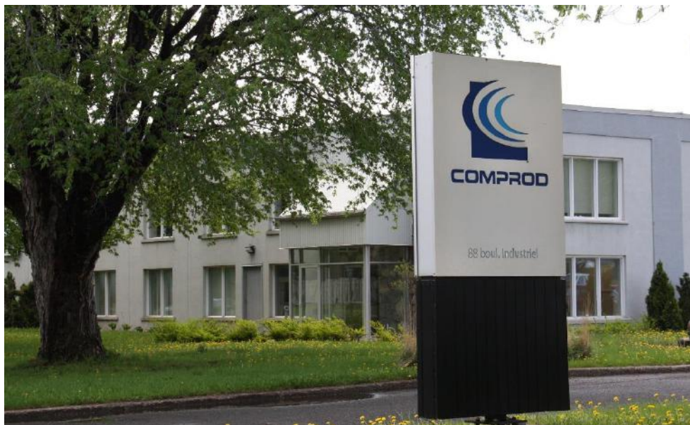
Comprod's Headquarter Facilities, Boucherville, QC, Canada
